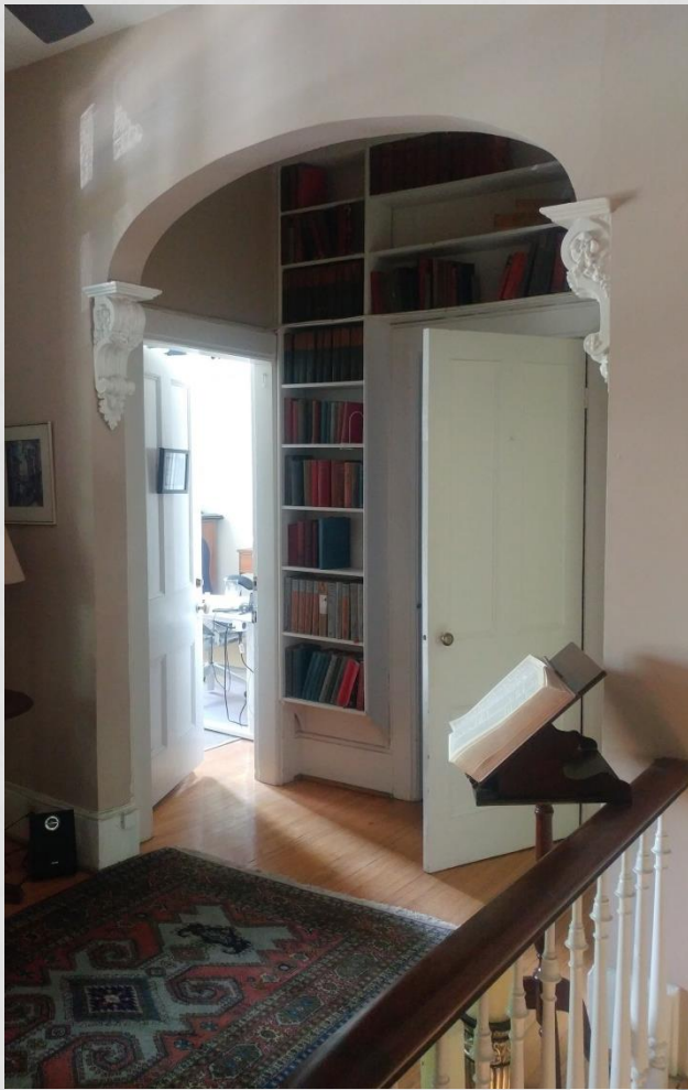
Interior plaster arch and corbel on second floor, 2018 (City of Guelph)
