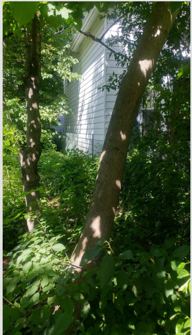
Temporary fence to be replaced by iron fence, 2018 (City of Guelph)
