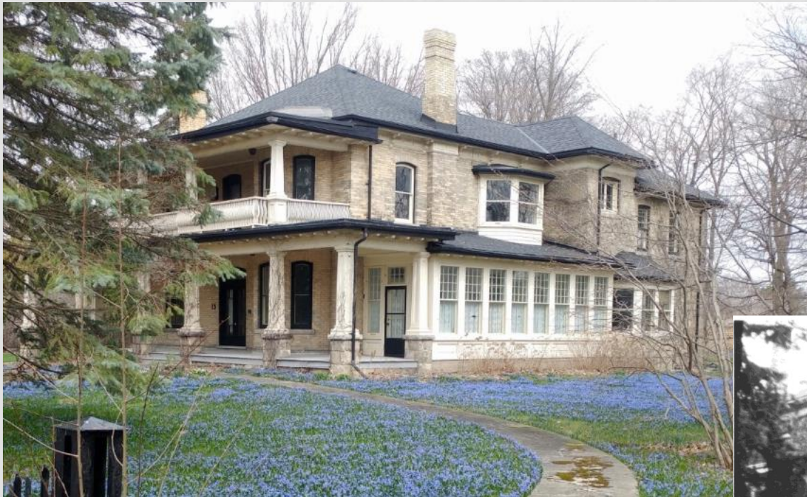
View from south, 2018 (City of Guelph)
