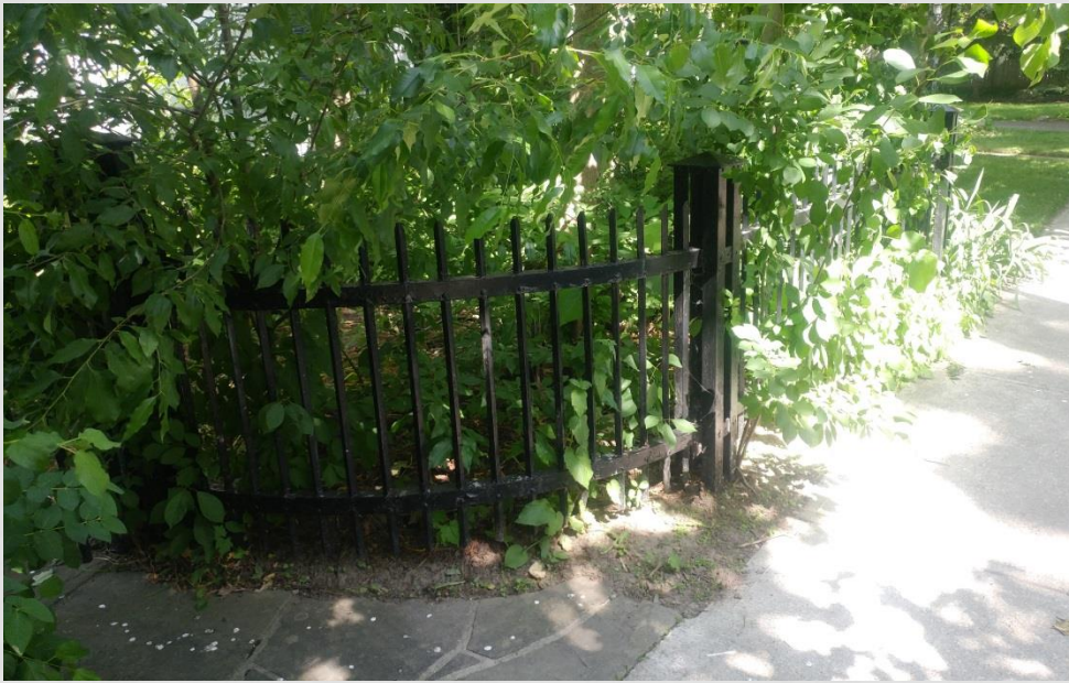
Curved iron fence at south gate, 2018 (City of Guelph)
