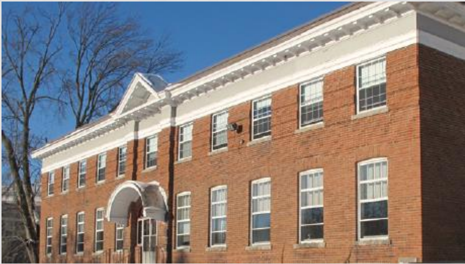
MacKinnon Building, 2013 (CHNER, ERA Architects Inc.)
