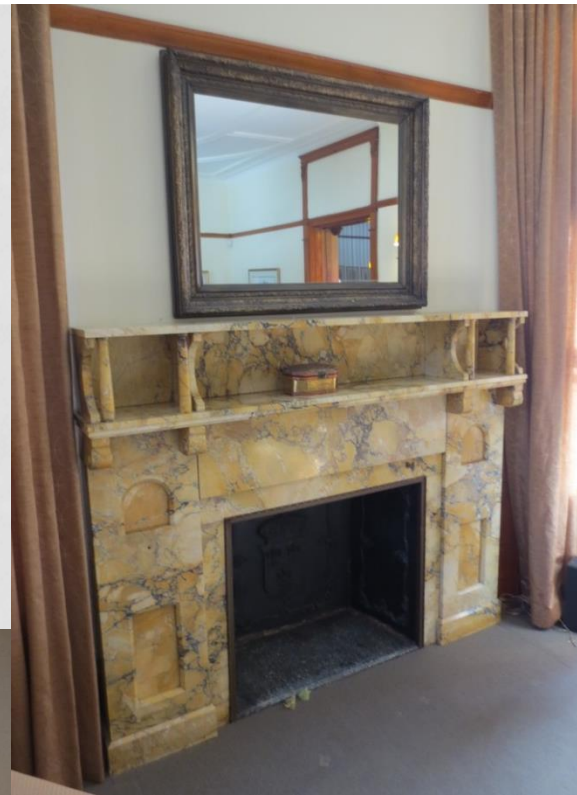
Riverslea Interior, 2018 (City of Guelph)
