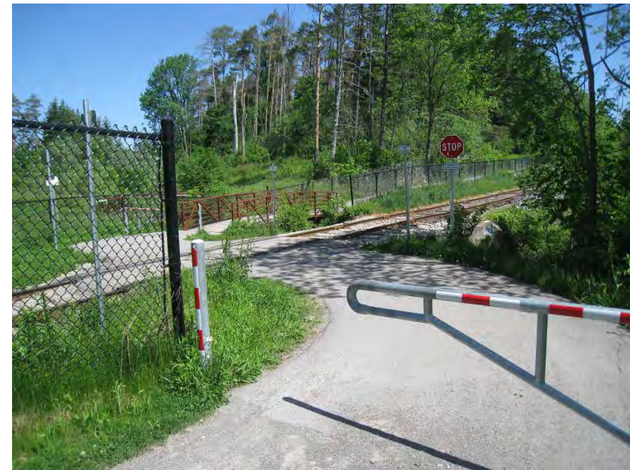
At grade railway crossing Hespeler, Ontario (2016)
