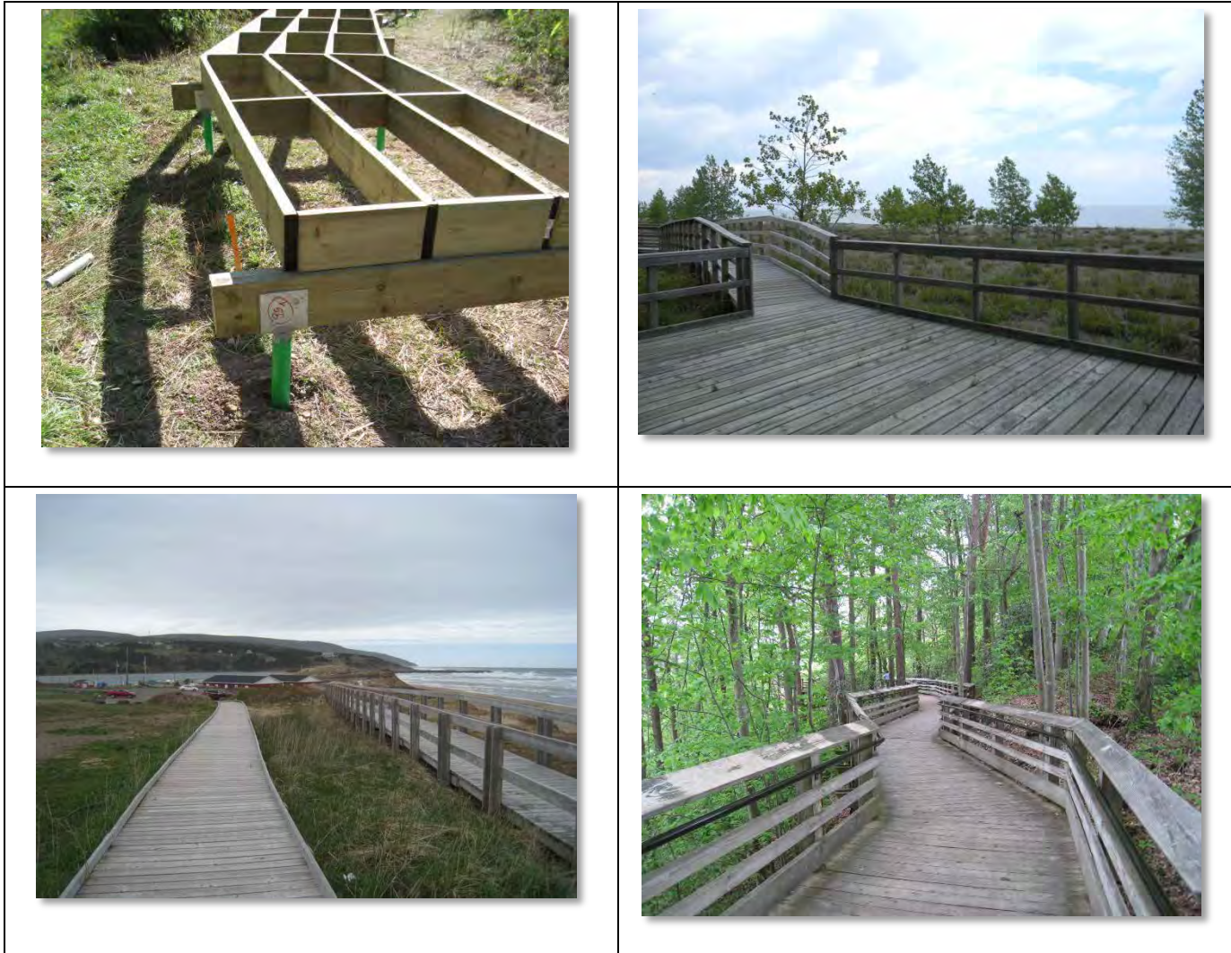
Figure 4.5: Boardwalks: top left – helical pier foundation Halton Hills Ontario, 2010; top right- Rondeau Provincial Park, Ontario over sensitive dunes, 2016, bottom left-low profile boardwalk with curb Inverness, Nova Scotia, 2017; bottom right through steeply sloped woodland, New River Gorge, West Virginia 2014
