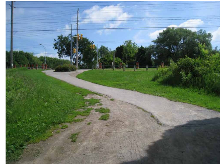
Existing Speed River Trail at Edinburgh Road, Guelph (2015)
