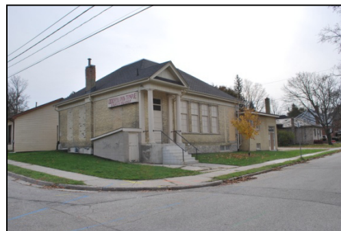
Blocking of window openings should be avoided
