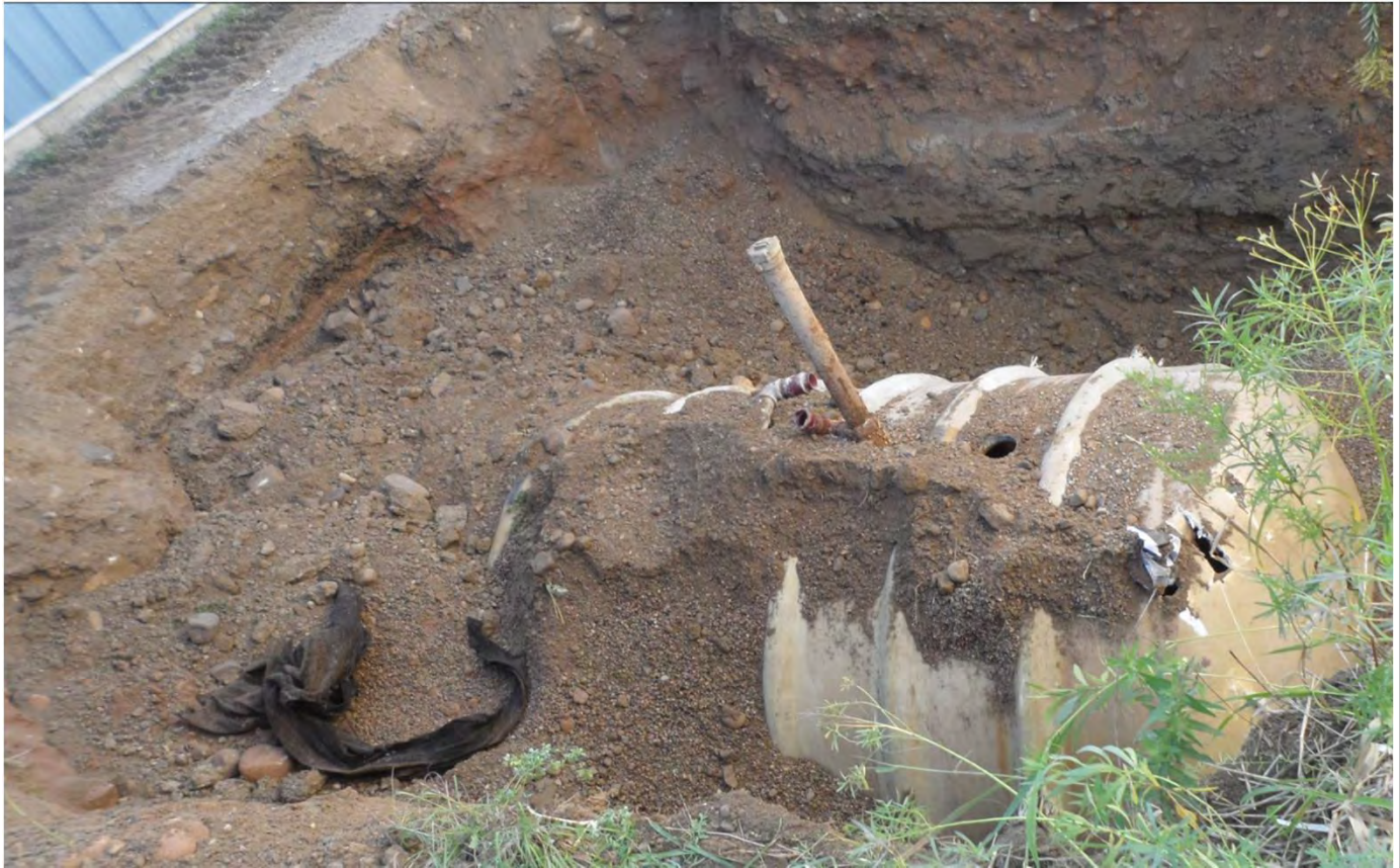
Photo 1 (top): Tank excavation area prior to field program. Pump and access port are observed.
