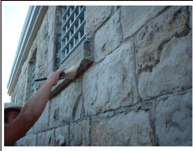
Photo.31: Brushing the joint to remove binder and to produce final finish
