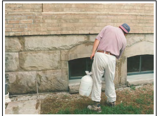
Photo.35. Curing repointed joints using mist-spraying techniques.
