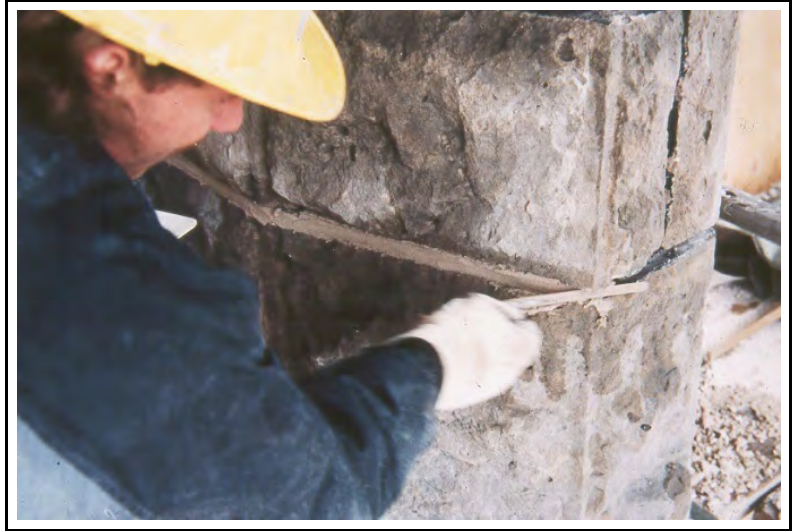
Photo.29: Applying the final layer of mortar
