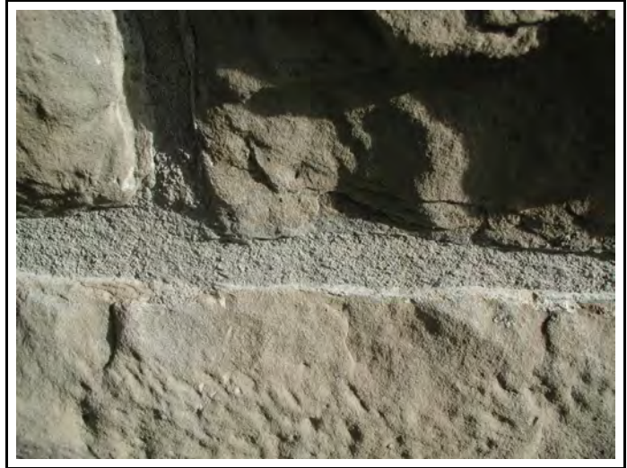
Photo.32. The finished joint
