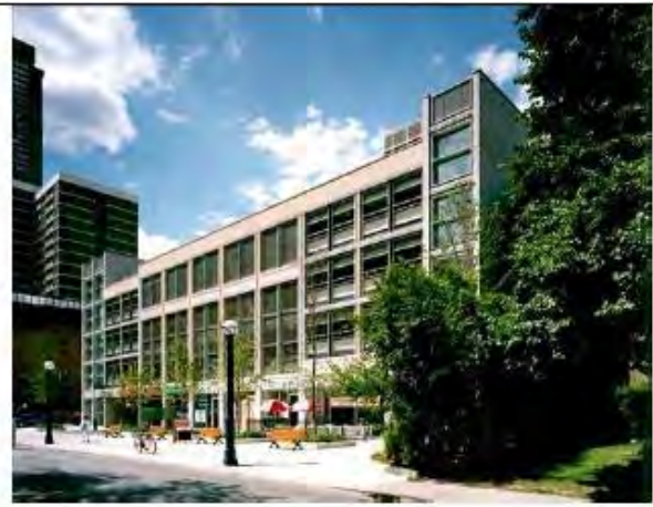
2. Parking garage with pedestrian amenities (good design)
