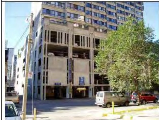
3. Parking garage with integrated residential development (good design)
