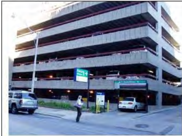
1. Parking garage with no urban design considerations (poor design)
