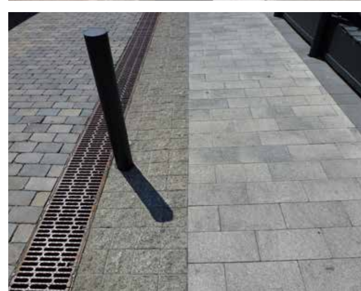
Figure 105 Precedents: Unique bollard elements may define areas for vehicles, with other forms of demarcation including mountable curbs and urban braille communicating transitions between zones.
