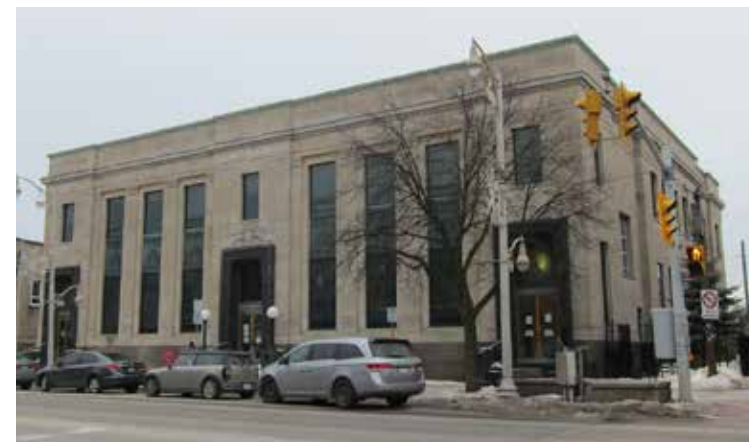
Figure 19 138 Wyndham Street North, street elevation
